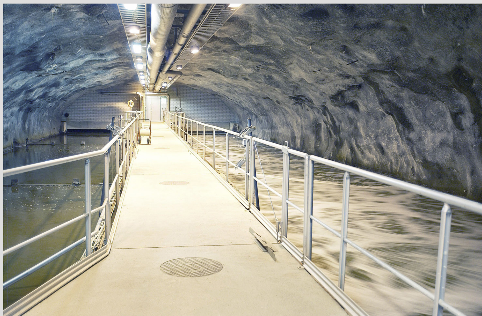
Fig. 1 Continuous emission monitoring at the bedrock wastewater treatment plant Helsinki Viikinmäki, Finland. Picture shows the denitrifying post-filtration unit. The underground area covers an area of 14 hectares, the above ground 3 hectares. Source: Sanna Alku, Helsinki Regions Environmental Services Authority (HSY).
